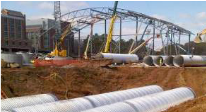
Construction photo of 1.4 Million Gallon Cistern (May 2010)
