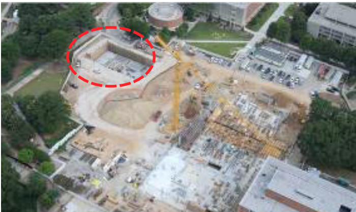
Construction photo of 1.4 Million Gallon Cistern (May 2010)
