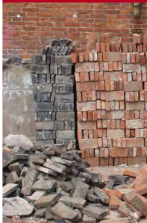
Salvaged bricks being sorted and stacked at Jian Ye Li.
